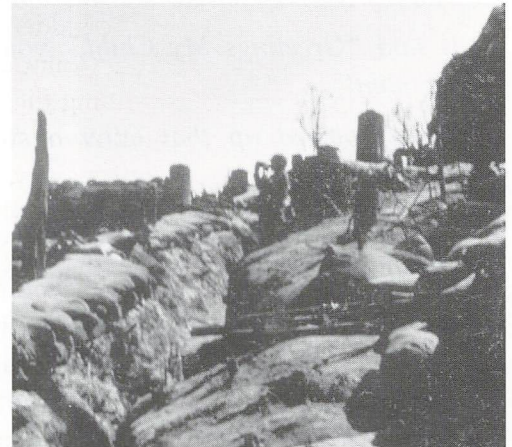
Trenchline in front of Dabney's CP, Hill 881S
